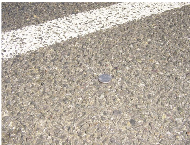
Figure 6-49: Photograph of I-80 Davis OGAC overlay
